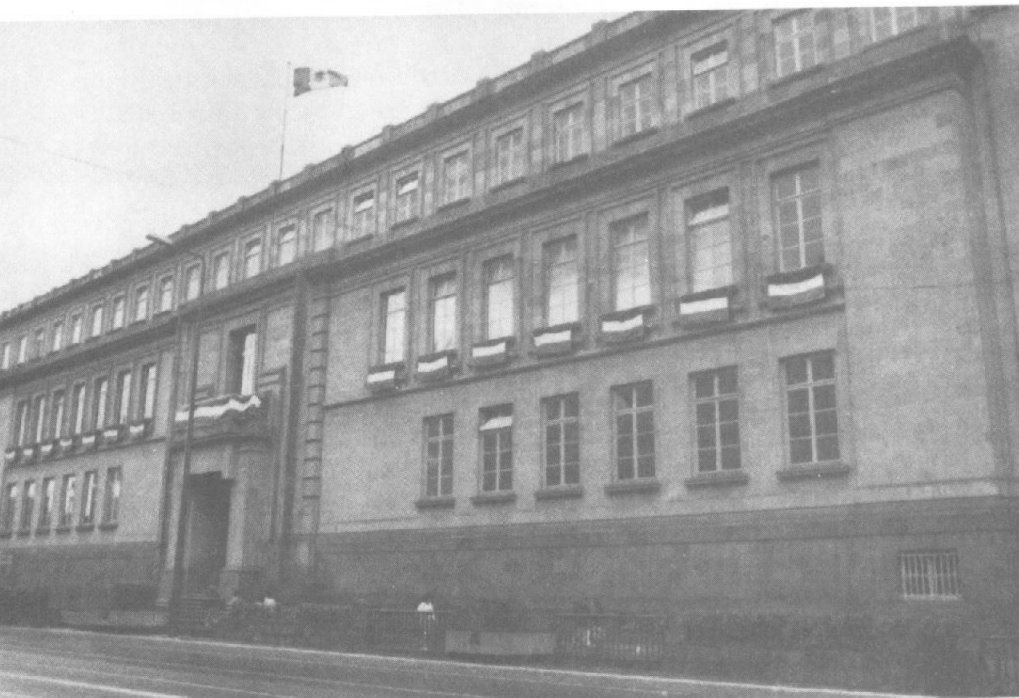
Congress building Courtesy Arturo Salinas Supreme Court of Justice building Courtesy Arturo Salinas
